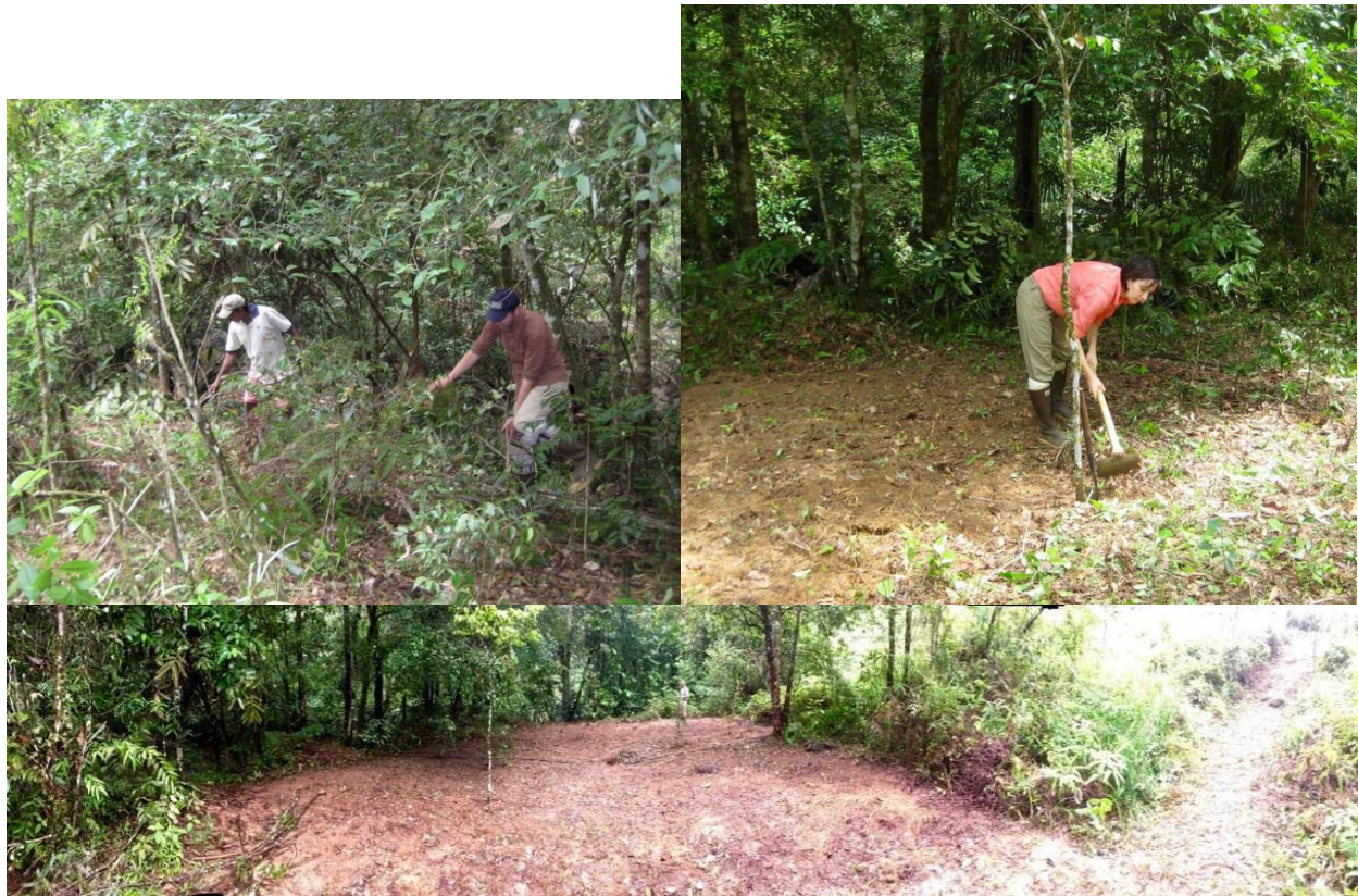
Figure 4. Creating a community nursery. A job well done. Logan and Somaratna starting the initial work clearing the brush. Laura hard at work with the mamatee (mattock). And the finished area ready for the creation of nursery propagation and germination beds.
