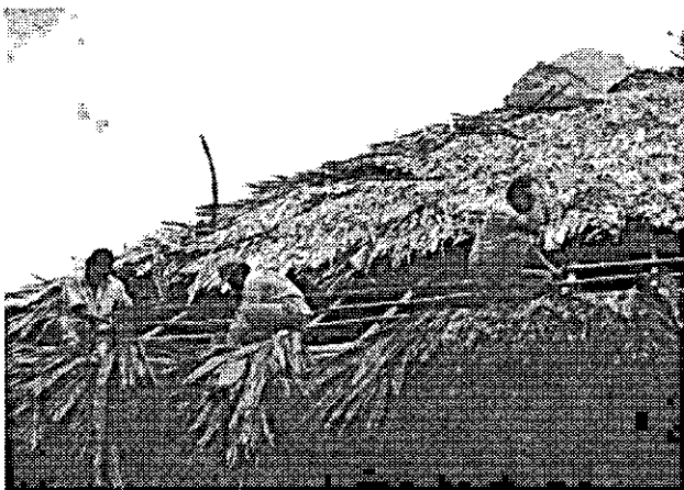
Figure 1. Belizean workers constructing a thatched roof.
