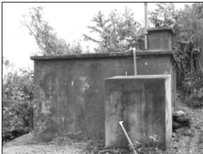
Figure 3. A storage tank built by one community's local ASADA. Water from a nearby stream is piped to this holding tank where chlorine is used to disinfect the water before it is distributed to households
