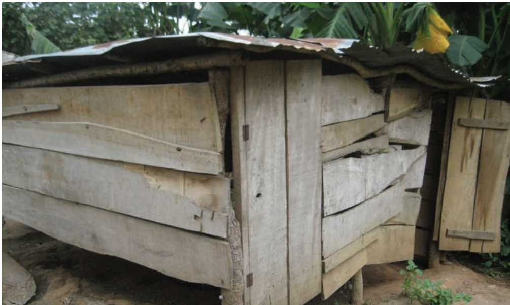
Photograph 3. A latrine constructed using only local materials in Aba Audu. CLTS encourages a variety of latrine construction options so that all members of the community can improve their access to sanitation.
