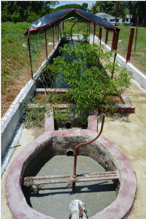
**Fig. 2.** Biodigester with round excrement tank innovation.
